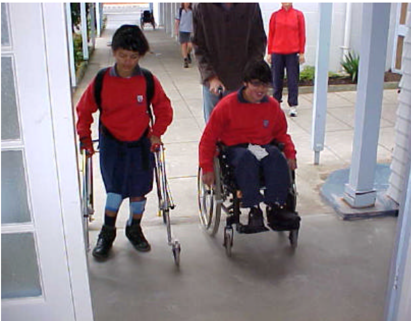
At long last, Taufa and Fleur with improved access. Two very happy students are the first to use the new front entrance ramp - one of seven currently being built/modified around the school.
